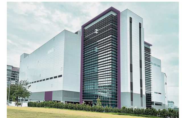
Singapore FEMS manufacturing facility
